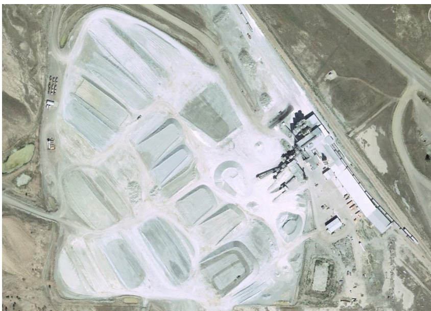
Figure 3 MTI drying pads, stockpiles and plant at Colony, Wyoming Source: Google Earth™
